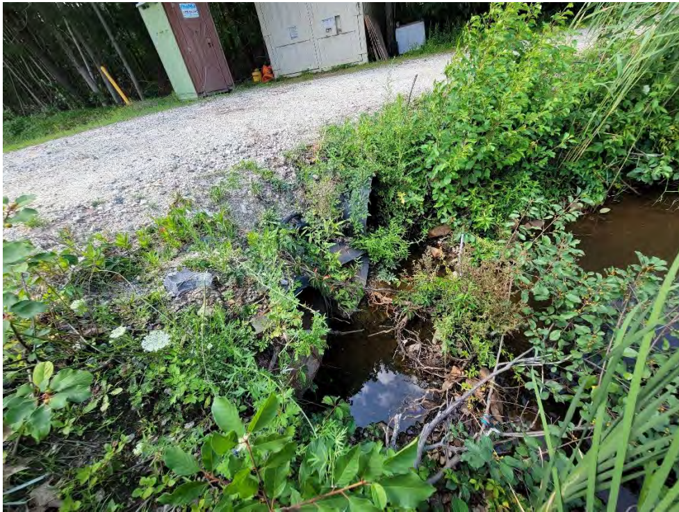
Photo 5. 3 culvert entry to the east of access road
