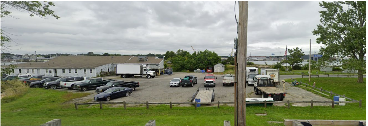
Operations Building and Grounds (Photo #10)
