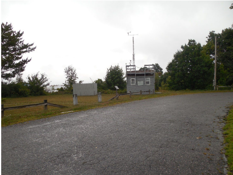
Driveway and Air Quality Monitoring Station (Photo #1)
