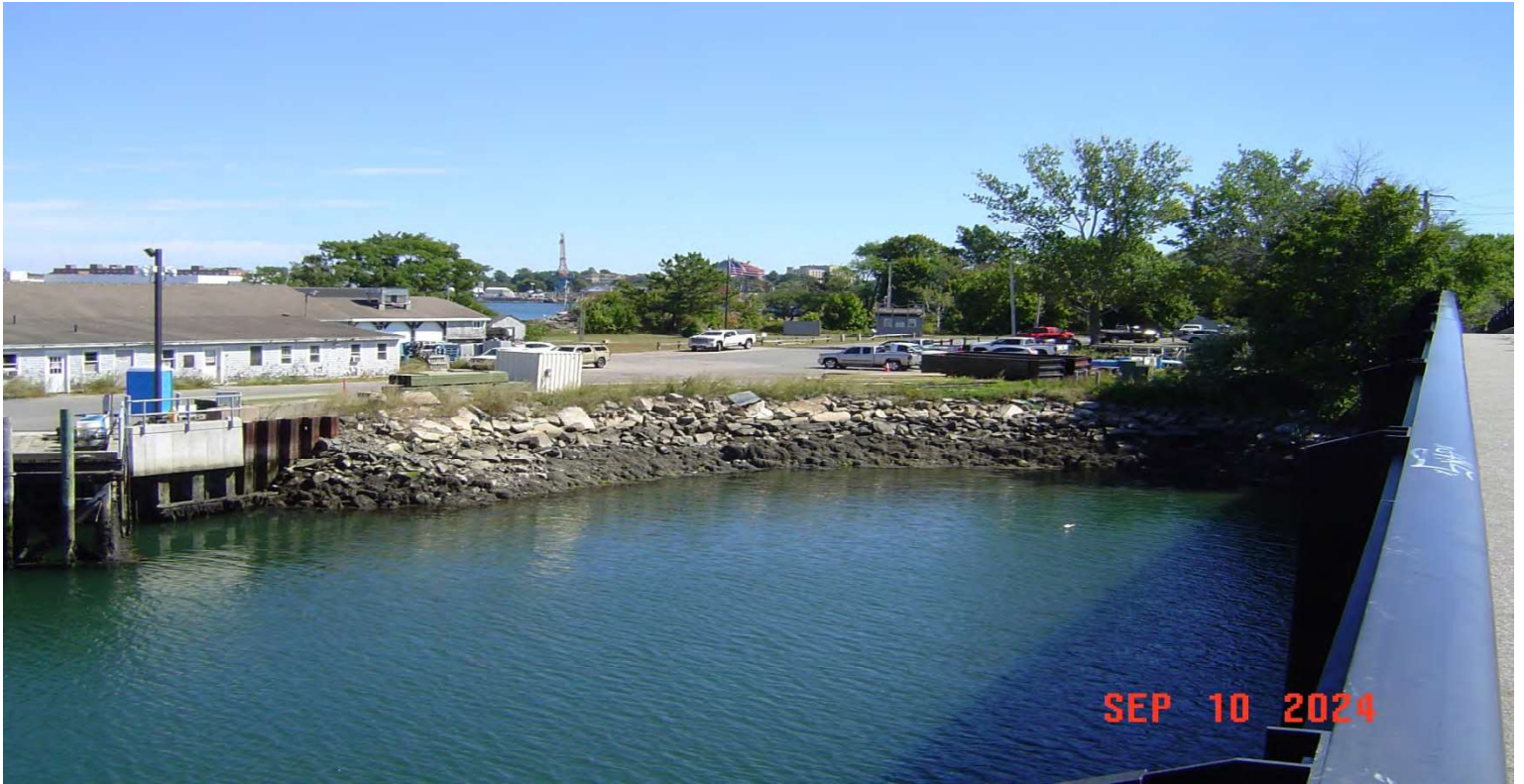
Image 1 – Looking easterly from the bridge over the river.
