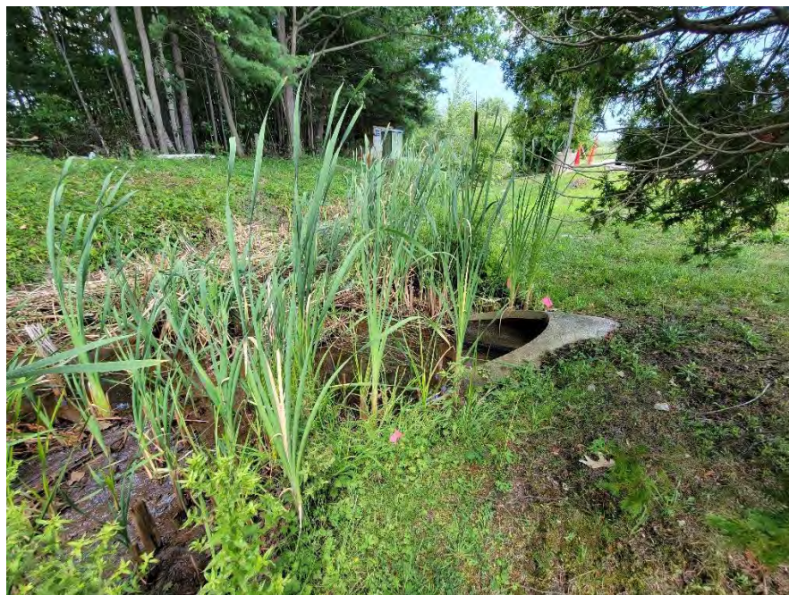
Photo 1. Culvert entry looking east toward access road
