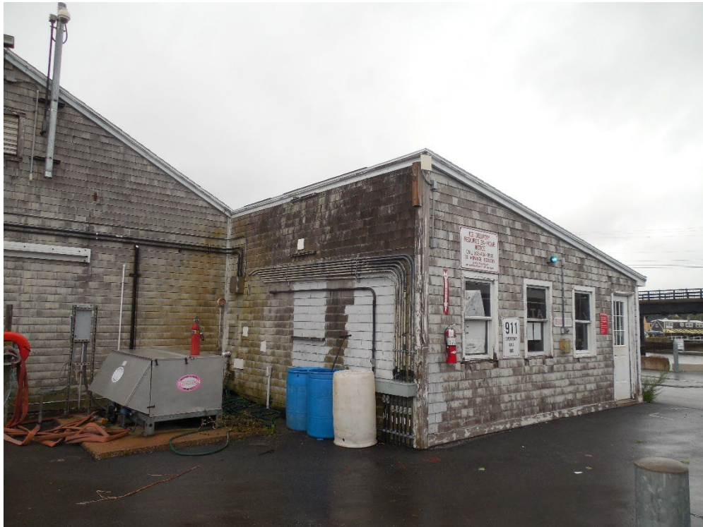
Operations Building – West elevation (Photo #8)
