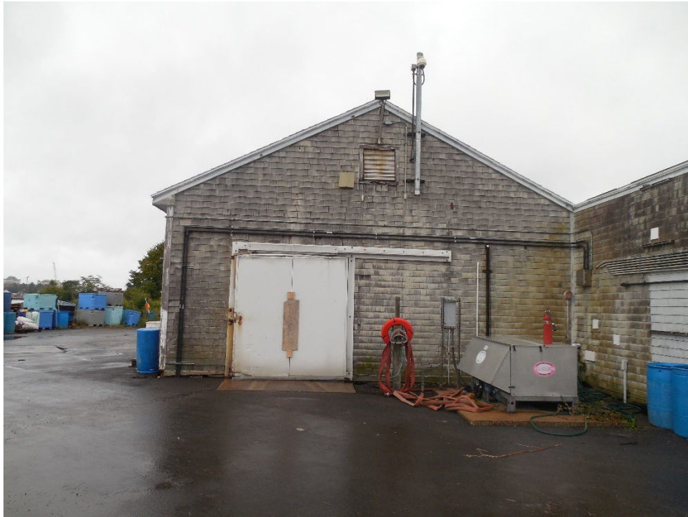
Operations Building – West Elevation (Photo #7)
